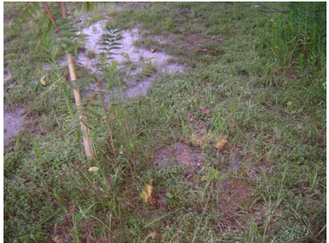
Photo 4: Water flowing from possible broken pipe at north end of site.
