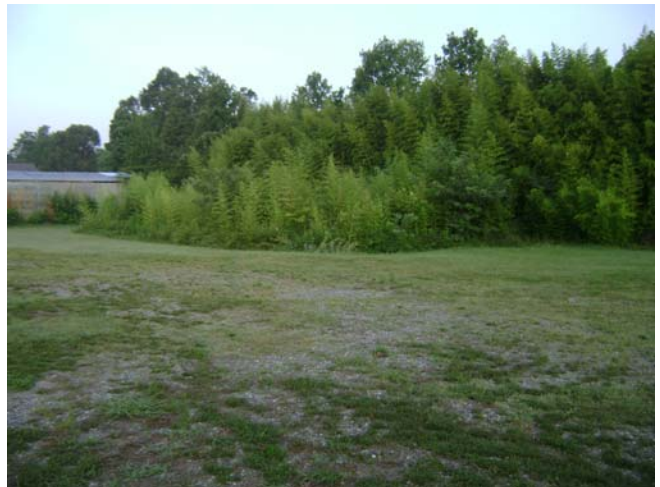
Photo 6: Looking west to existing storm dry pond overgrown with bamboo.
