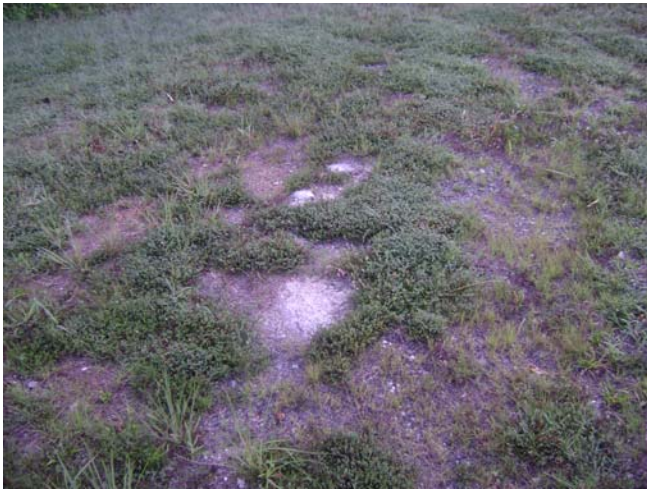
Photo 3: View of rock at ground surface at north half of the site..
